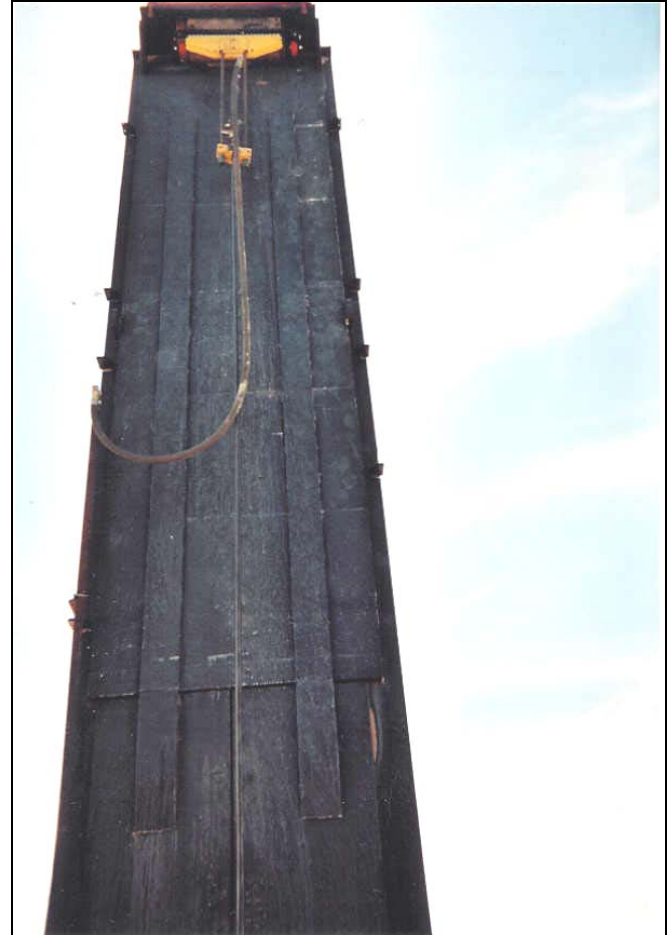
Figure 15: Surface Production Equipment
