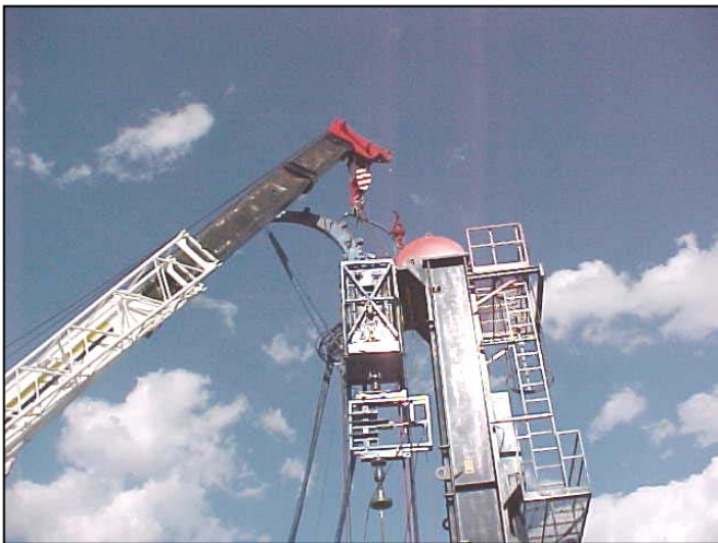
Figure 16: CTRS Installation Operation
