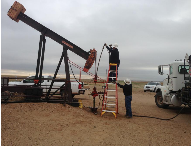
Figure 1 – Chemical Injection Setup.
